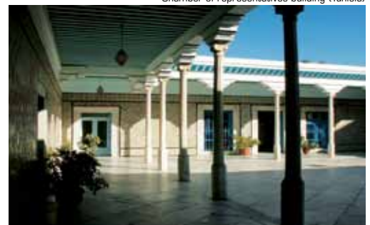
Chamber of representatives building (Tunisia)
