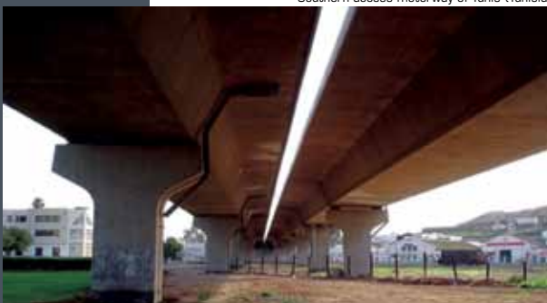
Southern access motorway of Tunis (Tunisia)
